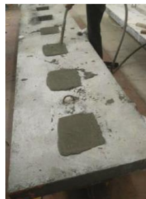
(c) Preenchimento das Shear Pockets com UHPC
