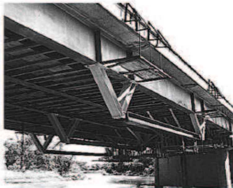
Figura 5. 10- Ponte Walnut Creek
